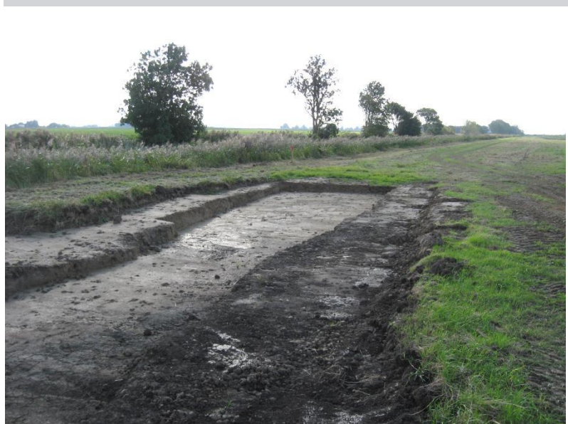
Photo: Constructed scrape
