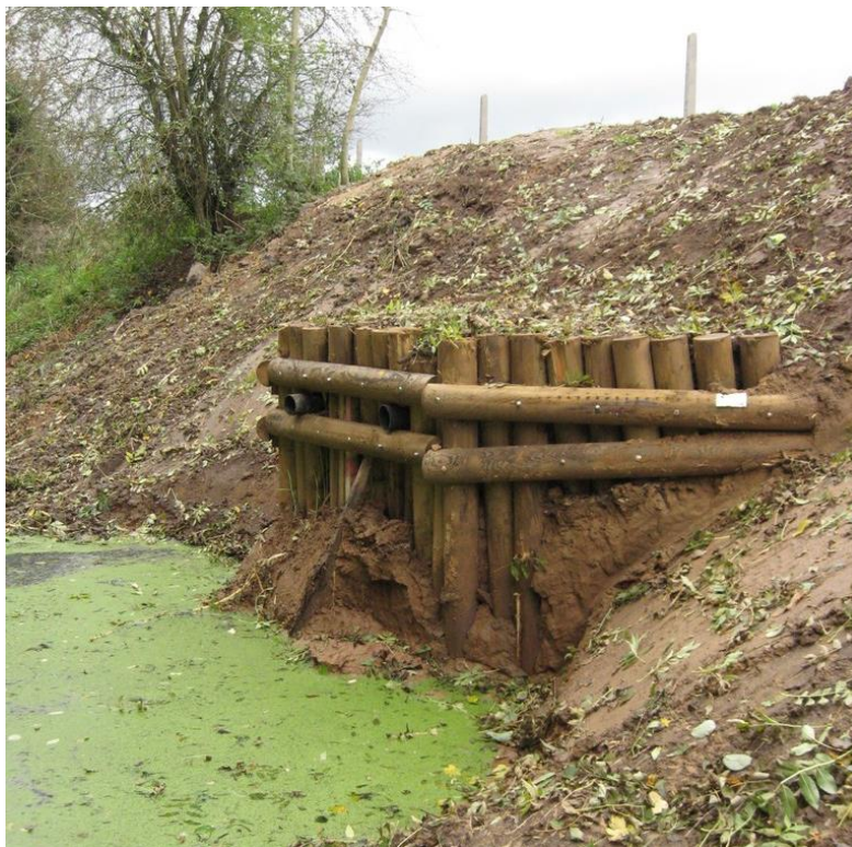
Photo: Constructed kingfisher bank
