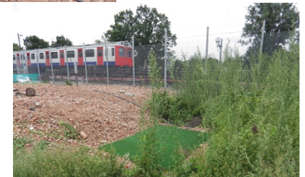
Swales with monitoring system
