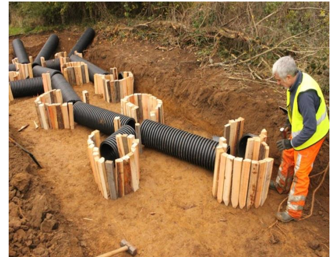
Artificial tunnels and chambers were created after liaising with badger experts.
