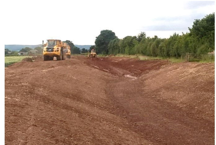
Creation of the flood defence channel
