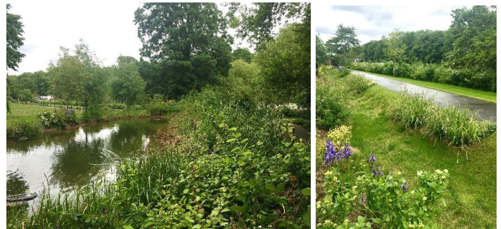
New pond, drainage hollows and public footpath created along the Thames.
