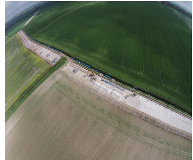
Part of the Pipeline Easement during Construction
