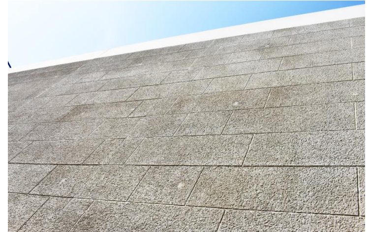
Figure 3. DWDR: Installation of Textured Concrete Surface at Wellington Navigation Channel.
