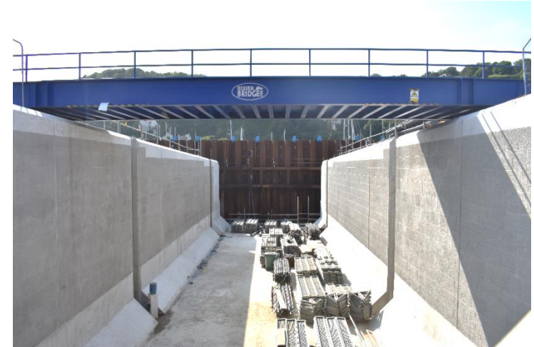
Figure 5. Finished Surface: Wellington Dock Navigation Channel
