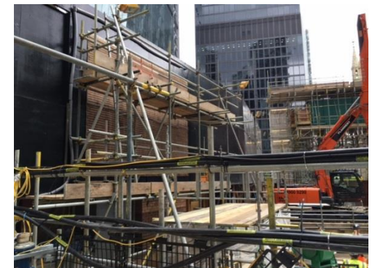
Under construction day 3
