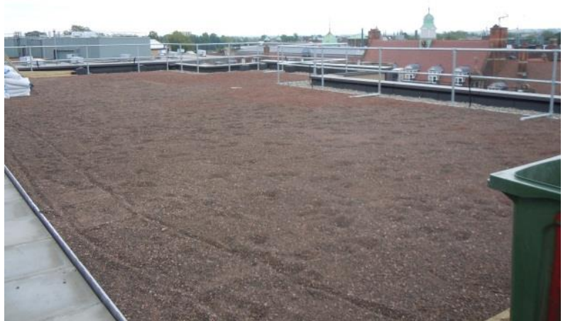
Photo: The expanse of the green roof
