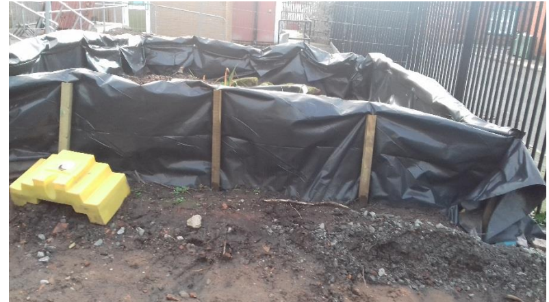
Temporary amphibian fencing
