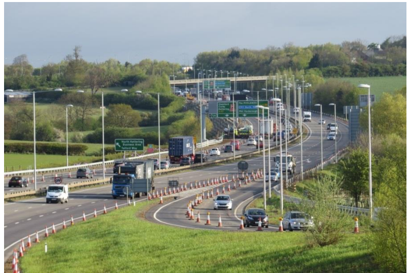
Photo: Road Overview
