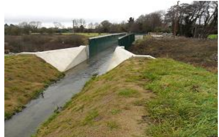
New aqueduct (upstream), December 2017
