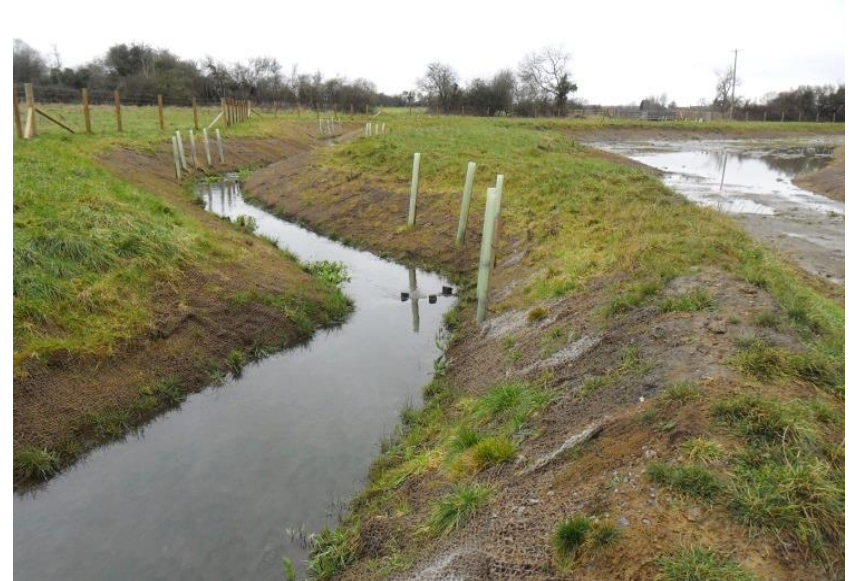
New channel and flood attenuation pond, December 2017
