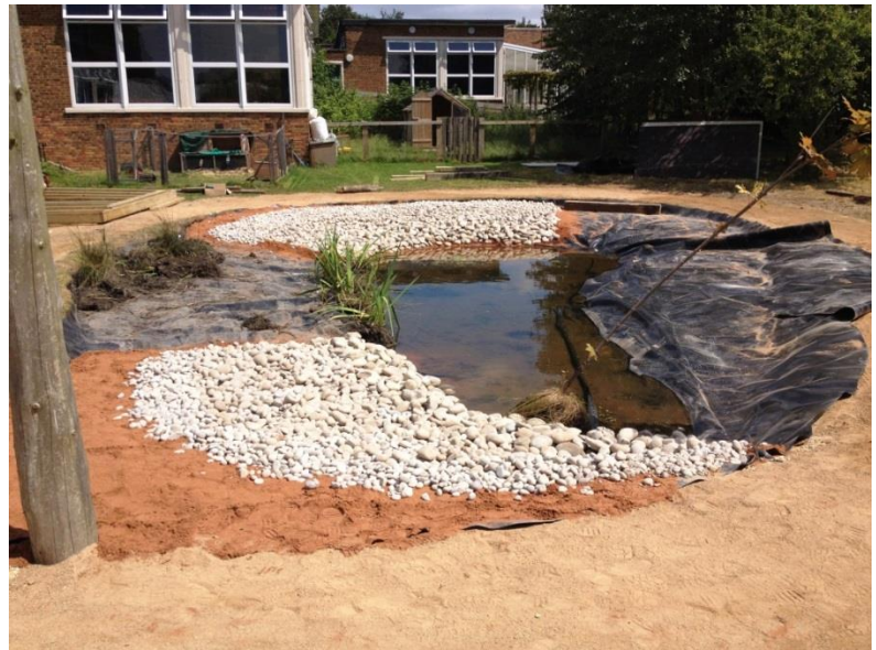
Photo: Pond under construction
