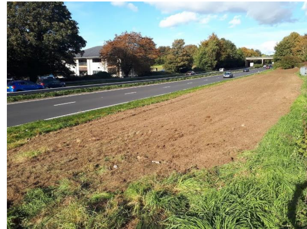
Ground preparation at one of the roadside sites
