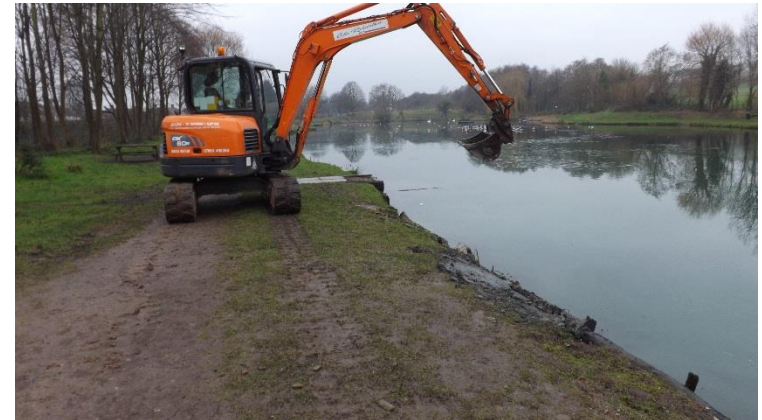
Pond bank stabilisation works
