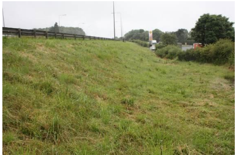
Photo: Early stages of reinstatement (2013)
