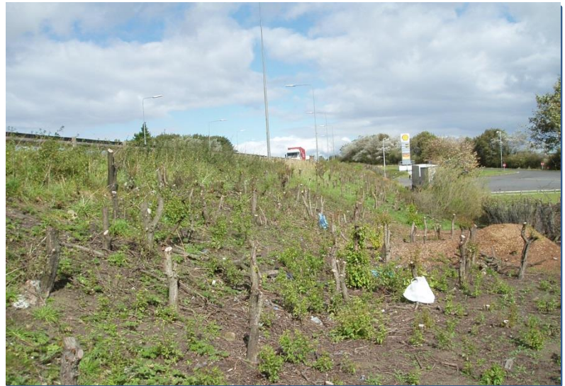
Photo: Site clearance (2012)
