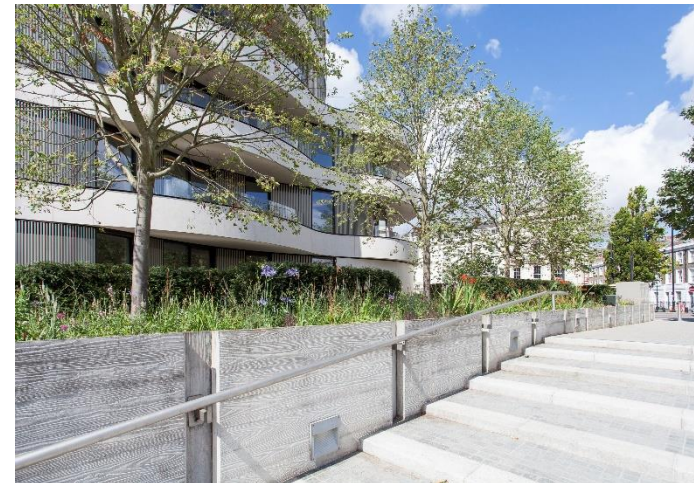
The semi-mature trees introduced to the site
