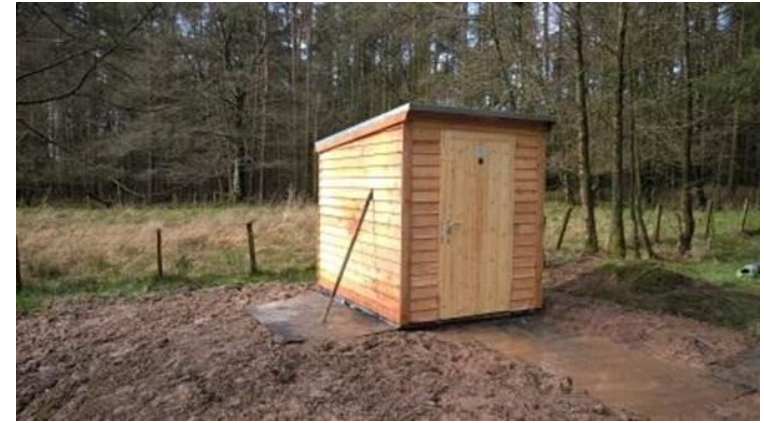
The erected building, awaiting access ramp
