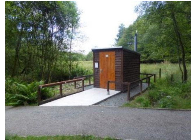
The completed structure
