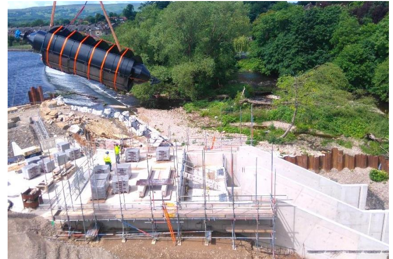
Archimedes Screw being manoeuvred into position
