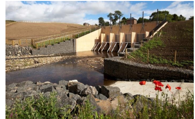
Dam inlet at the Mitford Flood Storage Area.
