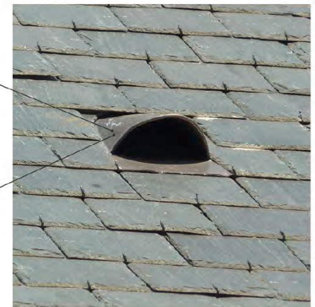
Access tiles to roof space similar to those used (Aspect Ecology)
