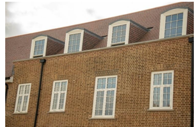
Mock dormer windows allowing access to roof roosting (S.Hughes)
