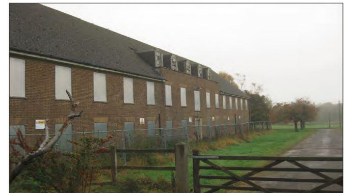
The Officer's Mess prior to renovation (photo: Aspect Ecology)
