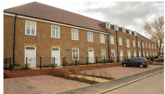
The Officer's Mess now completed (photo: S Hughes)
