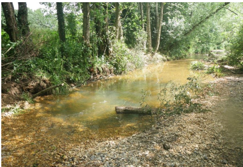
Photo: Completed top pool
