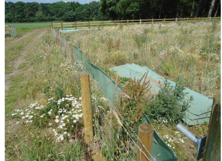
Reusable amphibian fencing implemented for extensive GCN clearance works
