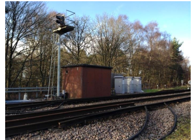
View of retained relay room next to railway. The signal box was located the other side of the signal from the relay room.
