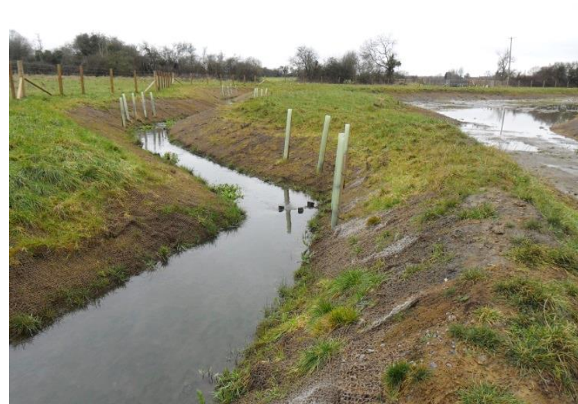
New channel and flood attenuation pond, December 2017
