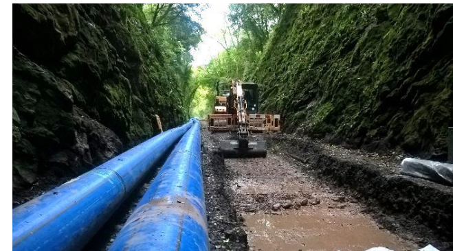
Preparation for pipe being laid in the tunnel
