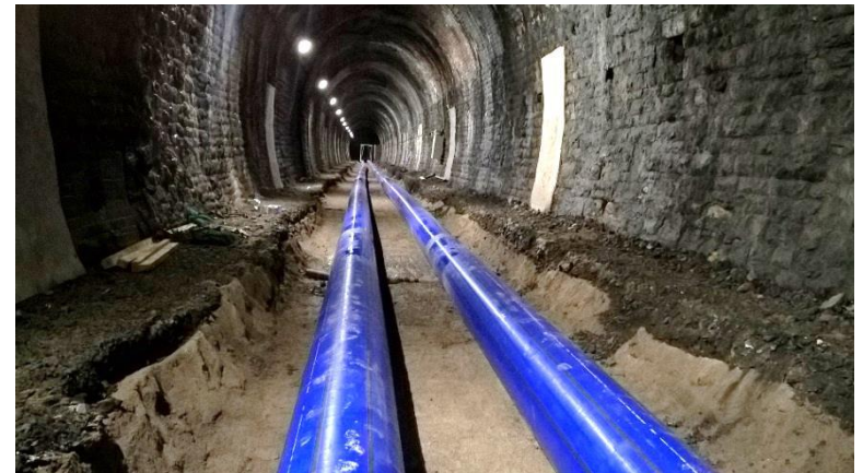
Pipe successfully laid in the tunnel
