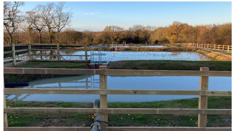
Clifton WwTW Integrated Constructed Wetland - Spring 2022
