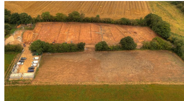
Aerial View of Clifton WwTW Site before construction
