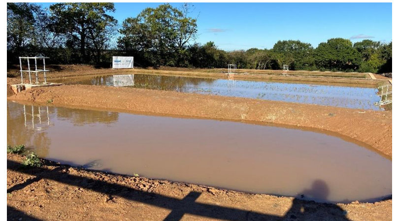
Clifton WwTW Integrated Constructed Wetland - ponds engineered to achieve the maximum amount of contact between the wastewater and the wetlands
