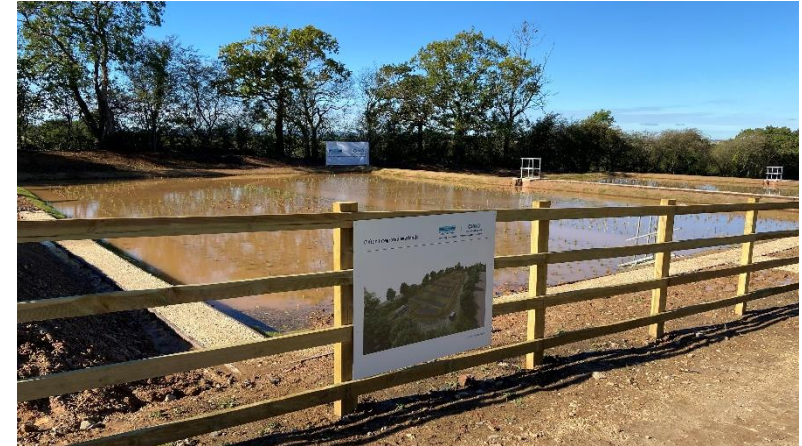
Clifton WwTW Integrated Constructed Wetland - Planting completion
