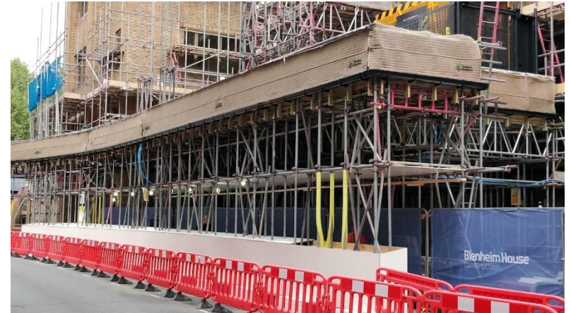
Vertical Meadow Wrap following installation
