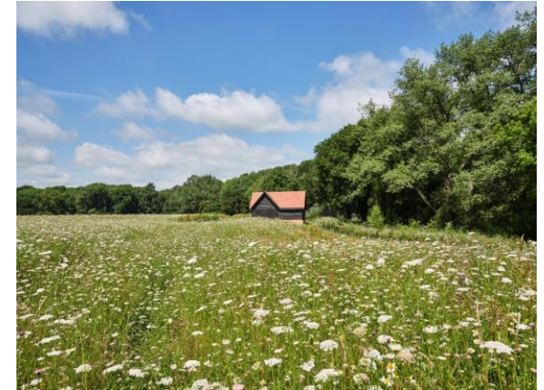
Swanbourne Bat Structure sat in an ECS, adjacent to mature woodland:
