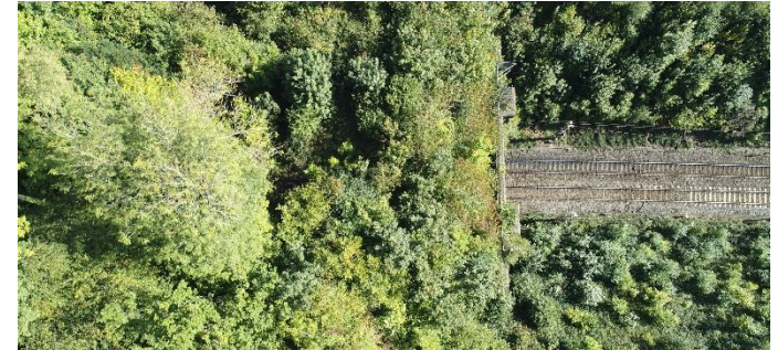
The Network Rail lineside estate
