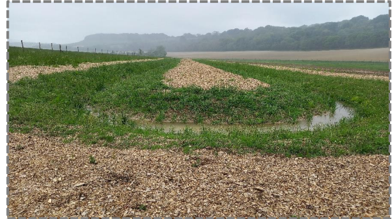
Vegetated swale adjacent to main wetland, with woodland planting along mulched margins (Meon Springs)
