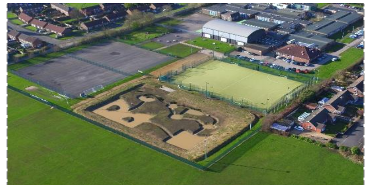
2015: Aerial view of the wetlands after initial construction.
