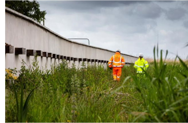
Habitat shelved installed on concrete walls to create microhabitats
