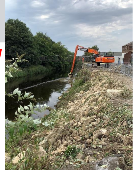
Previous / before photo of the bank at the Tannery site.
