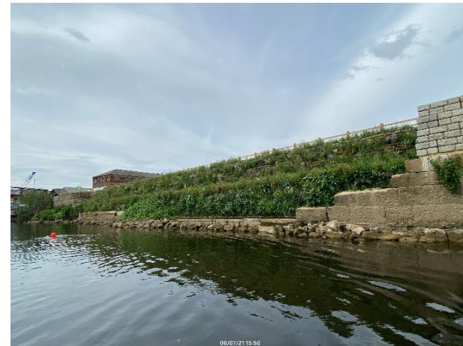
Full earth embankment photo
