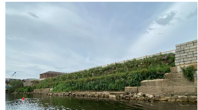
The vegetated, flowering reinforced earth embankment at the Tannery site
