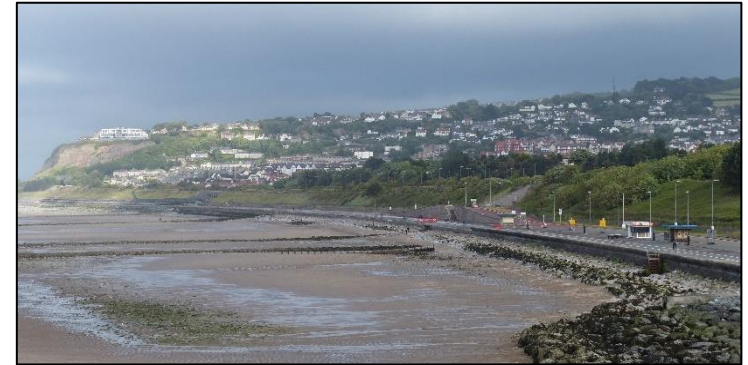
Looking North-East from Porth Eirias across Scheme area (prior to construction) – Mott MacDonald Ltd
