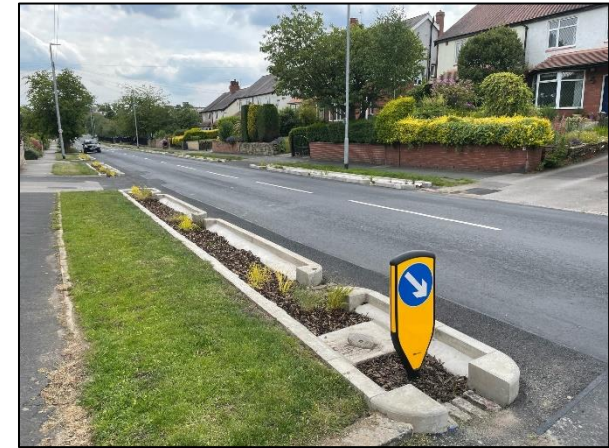
Rain gardens convey surface water via a gravity system for 190m along each side of Roman Avenue.
