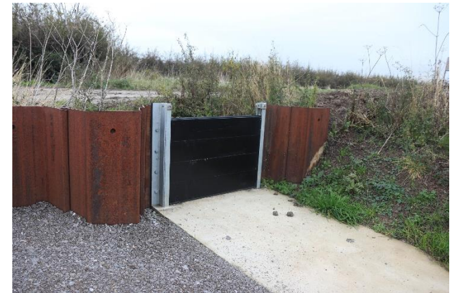
Flow control structures constructed.
