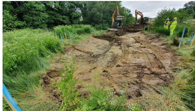
Pond creation using excavators (Photo By Cormac)
