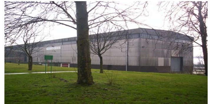
Main papermill building prior to demolition
