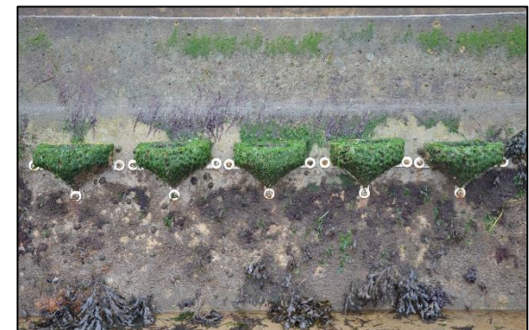
The seawall at Sandbanks following rockpool installation 6 months on.
