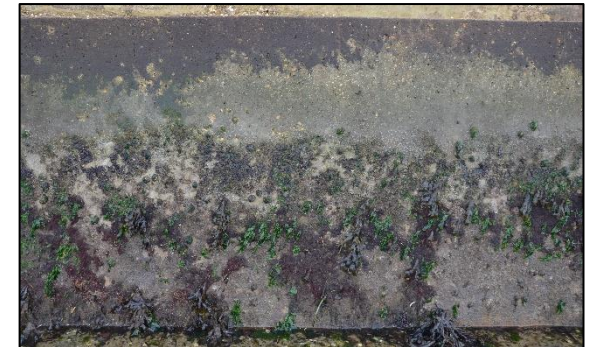
The seawall at Sandbanks prior to installation.
