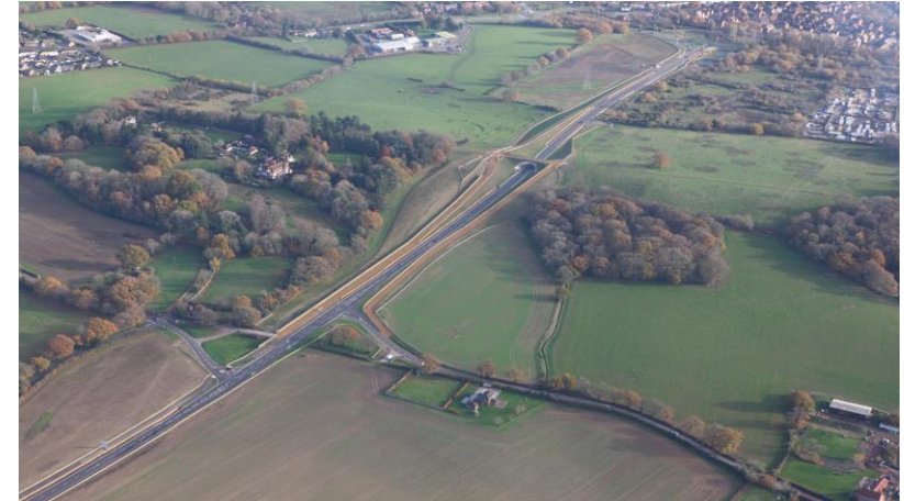
Plane imagery of the new ACRR, looking south along the alignment. The Green Bridge is visible, linking Spring Copse, (immediately west/right of the alignment) the Arborfield Court Woodland (immediately east/left of the alignment). The Green Bridge maintains the line of the PRoW (visible in image), with the ACRR dug into cutting at this point of the alignment.
