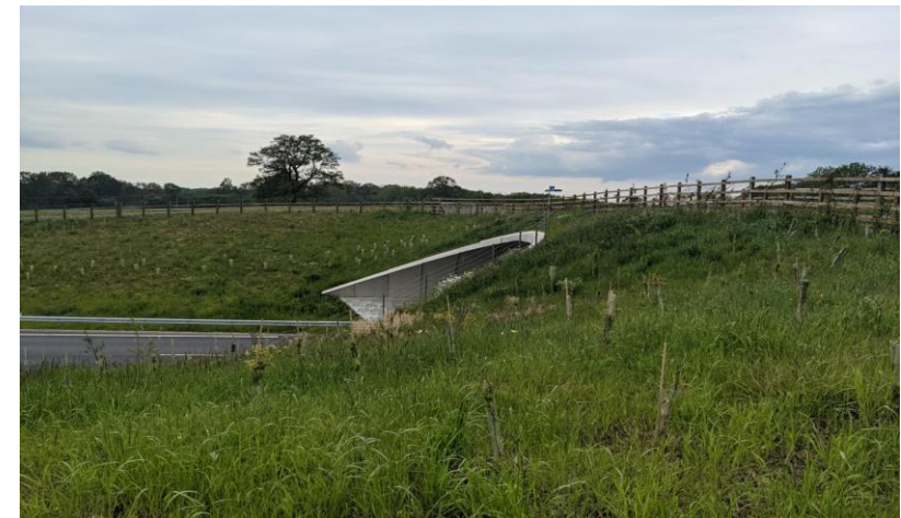
Green Bridge at ACRR with newly installed planting – southern span, looking west
