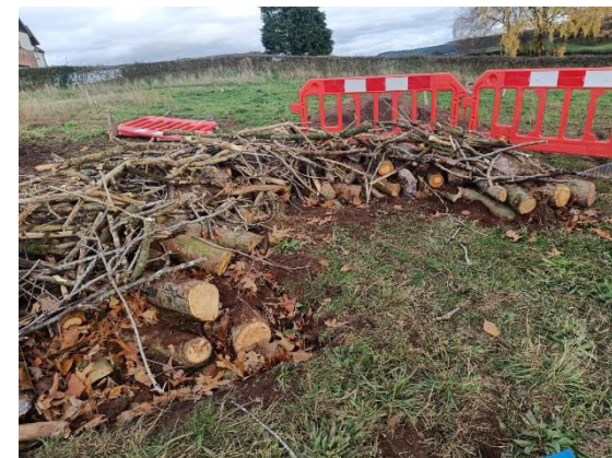
Creation of reptile hibernacula by EEW contractor from HP29 donated timber.
