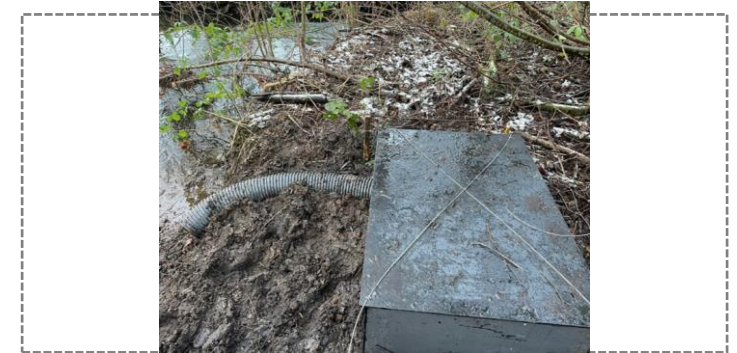
Process of installing artificial otter holt at riverbank
