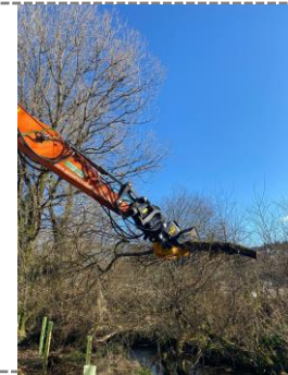
Clearing the riverbank
