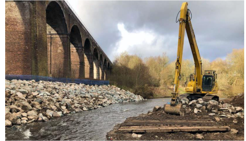
Rock Armour installation during emergency works
