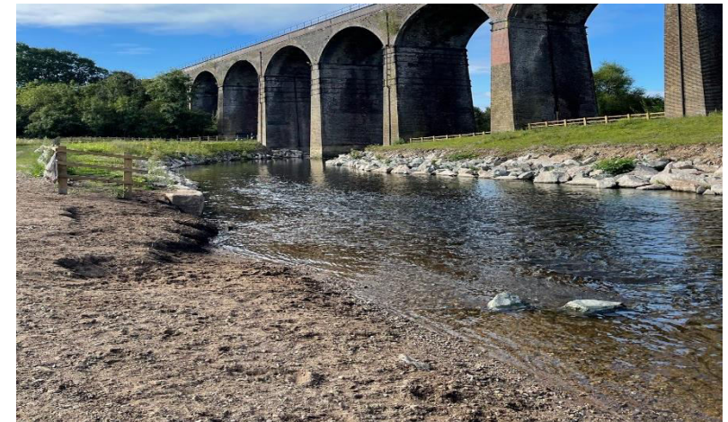
Completed works showing the beach for locals
