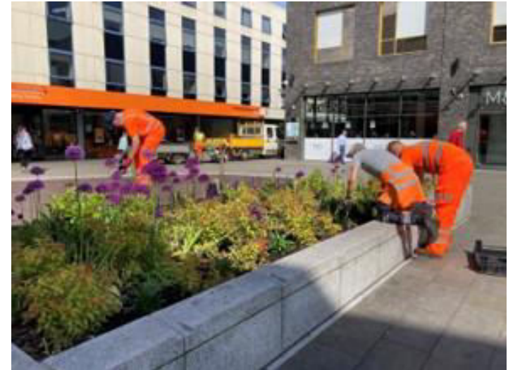
Planting in progress in John Frost Square
