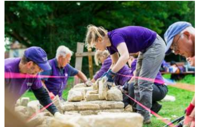
Drystone walling with volunteers, 2021. © The Parks Trust.
