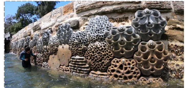
The Living Seawall, 6 months after installation at Sawmillers Reserve, McMahons Point, Sydney, Australia
