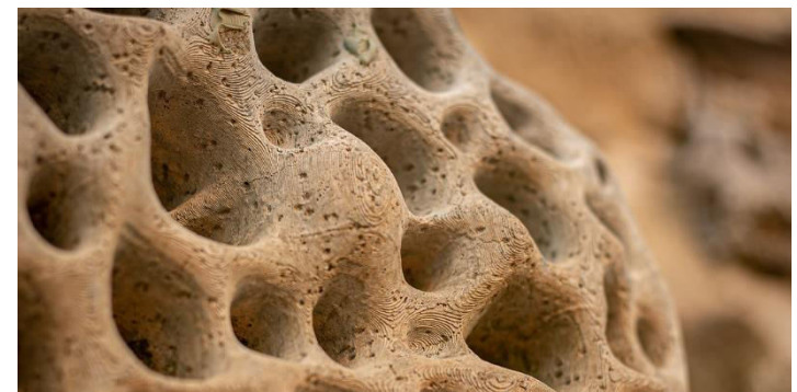
Living Seawalls panels are designed to mimic features of nature
