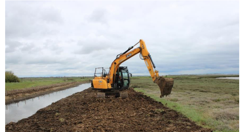
Removal of the south-east embankment through the process of managed realignment to create new saltmarsh © Katherine Gilchrist
